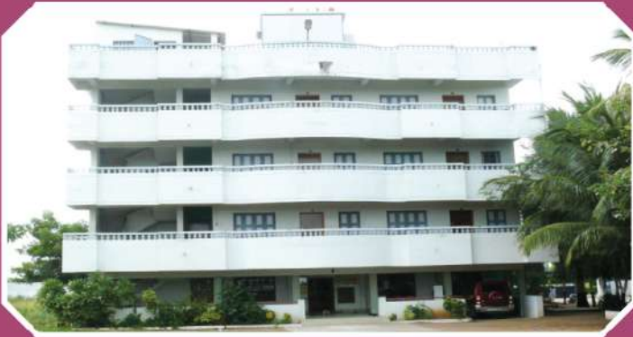
Administration & Hostel Block
